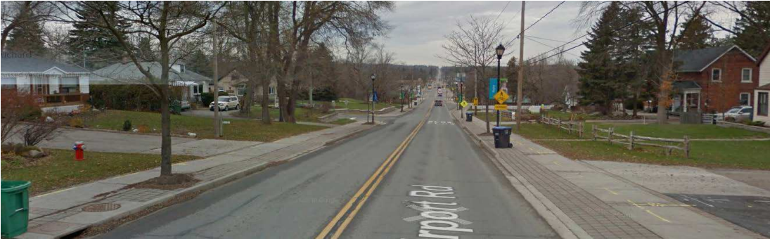
Airport Road from Hilltop Drive to Walker Road
